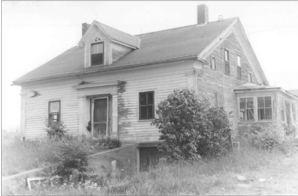
Dean Homestead. Historic Sites and Structures Survey: Addison County (Survey No. 112-5)
